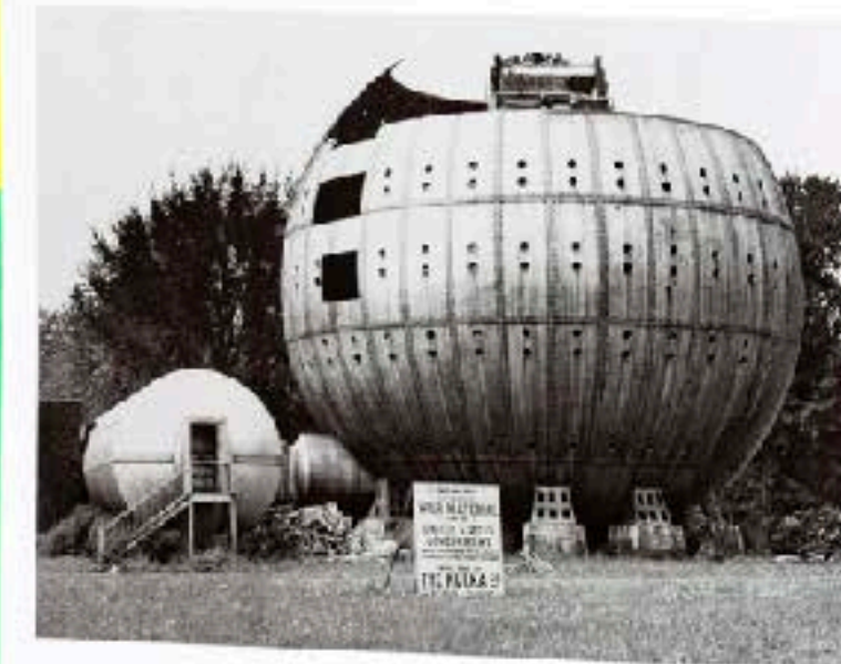
The Cunningham Sanitarium sphere during construction by Orval Cunningham for the war effort, 1917. Photograph by Walker Krieger. Cleveland: 1928 Collection.
